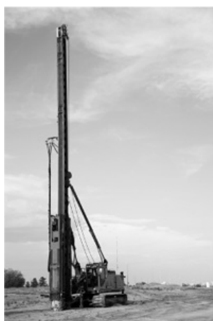
Figure 4.5: Photograph of a pile driver.
